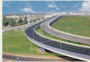
Construction of Road, Bridge and Railway Line
