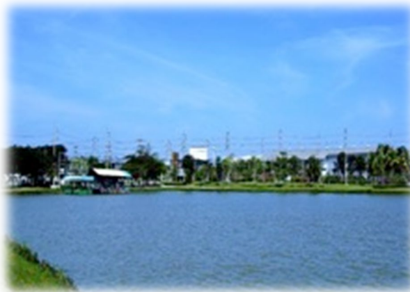
供水廠及儲水池 Total Raw Water Supply: 34.7 million m 3
