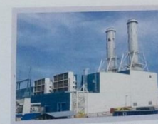
4. Small Power Plant
